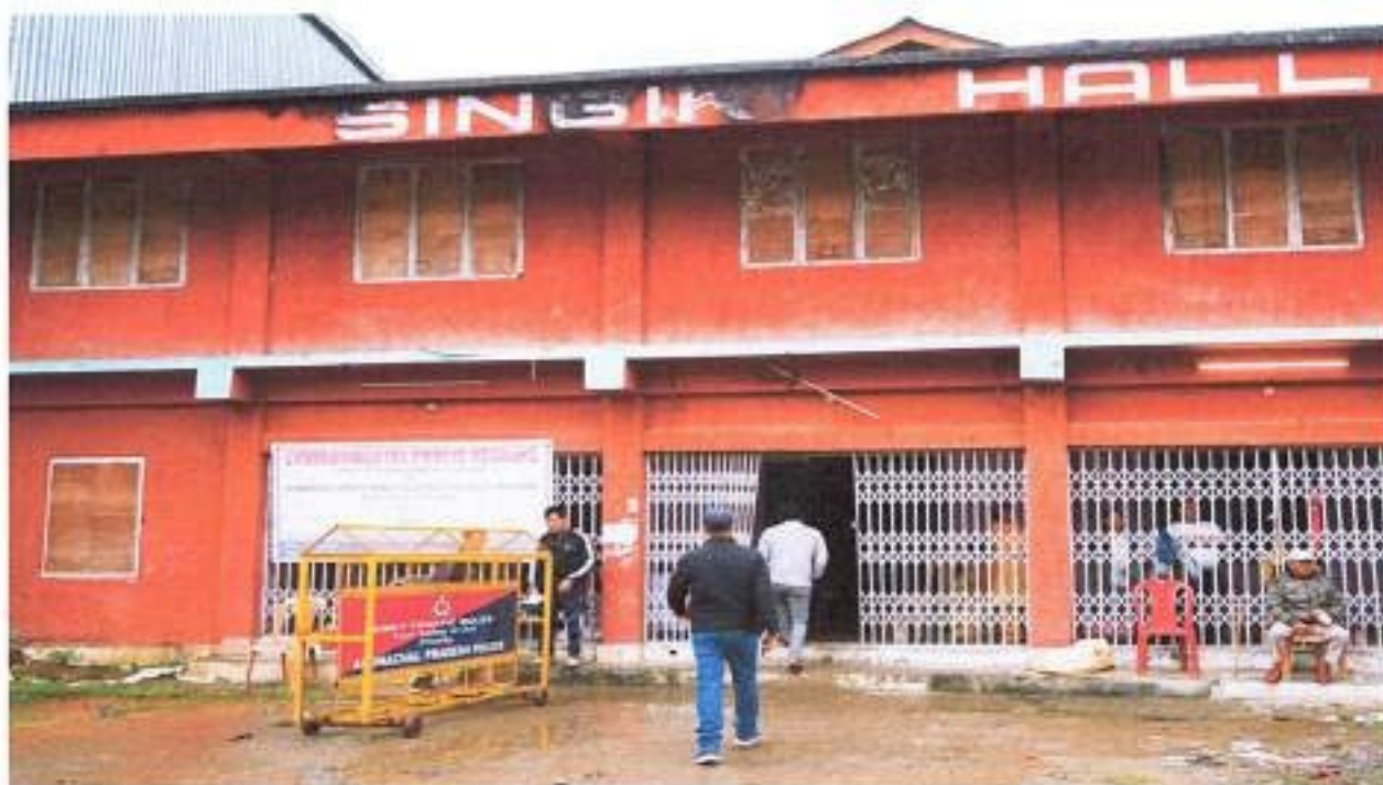
Picture-1: Singik Hall, Daporijo, Upper Subansiri District, the venue of Environmental Public Hearing of Subansiri Upper Hydro Electric Project (1605 MW).
